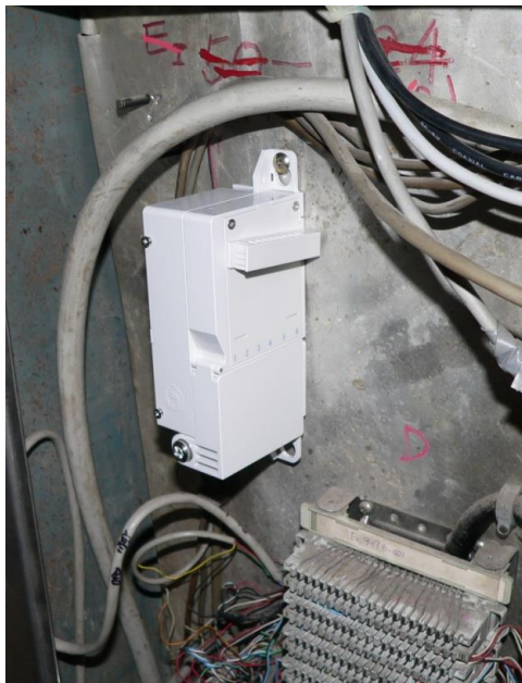
WIM-OCDB-E type is installed in indoor distribution panel, chief/ main box or appropriate location for fiber splicing
